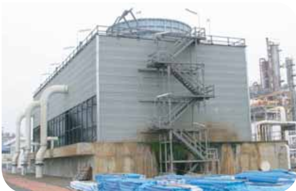
:: Petronas VCM Reconstruction, 13500 m 3 /hr (3 cells).
