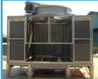
HDG Steel Structure
